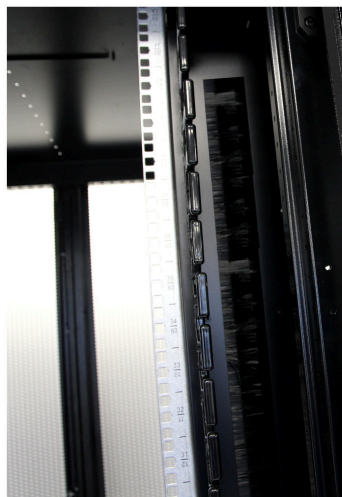
Airflow Management Baffles
