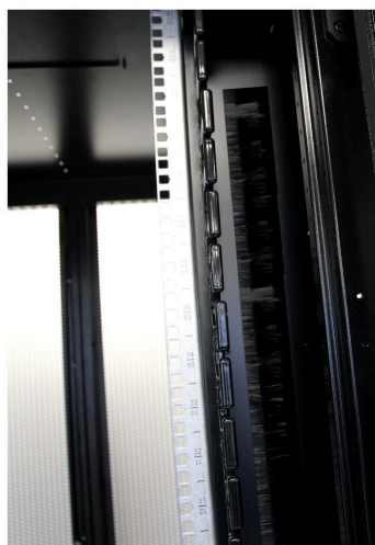
Airflow Management Baffles
