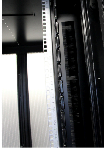
Airflow Management Baffles
