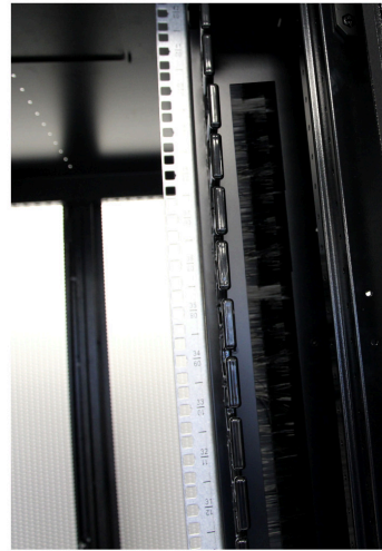
Airflow Management Baffles
