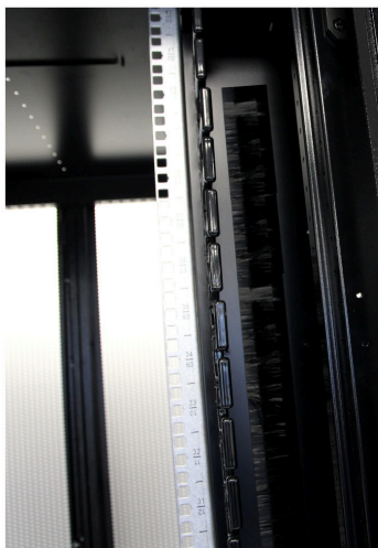
Airflow Management Baffles
