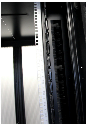
Airflow Management Baffles
