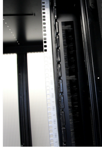
Airflow Management Baffles
