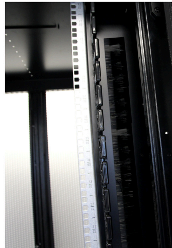
Airflow Management Baffles
