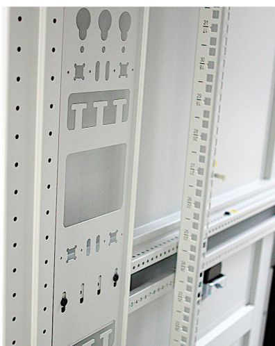
PDU mounting Cable Tray
