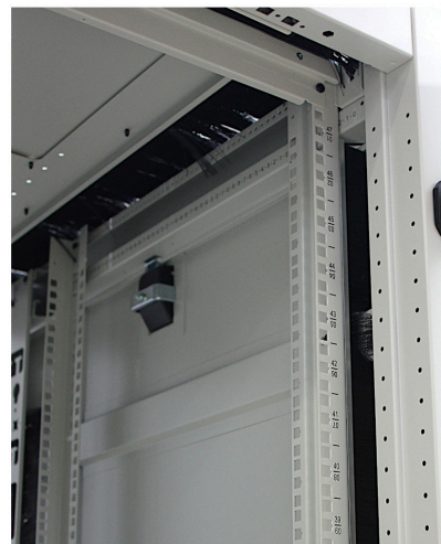
Airflow Management Baffles
